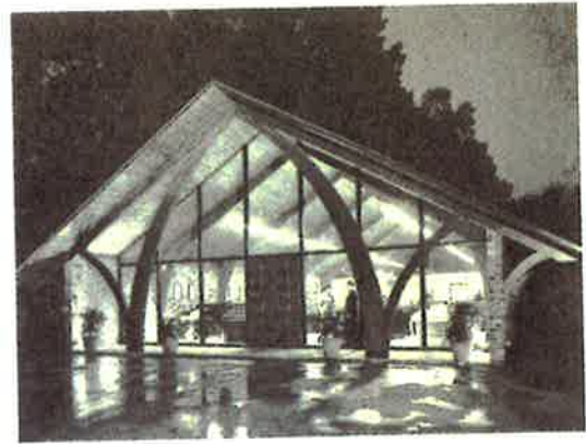
Fig. 1-10. The appealing design of this commercial building uses laminated structures to solve a technical engineering problem. (Southern Pine Association.)
