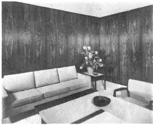
Fig. 1-5. Brazilian rosewood, one of the most sumptuous woods in the world, is used lavishly in the plywood panels which line the walls and conceal the built-in closet areas in this executive office. (United States Plywood Corporation.)
