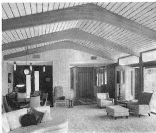
Fig. 1-8. The interior of this home is made most interesting because of the laminated ceiling and roof supports, and the beautiful wood ceiling and wall treatment. ( Weyerhaeuser Company. )
