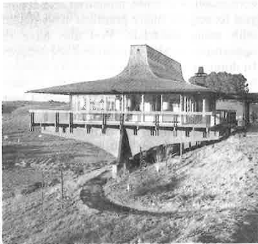
Fig. 1-7. This imaginative, dynamic, cliff-hanging house has won many awards for the wood products industries because of the ingenuity in the use of laminated supporting structures, and the interesting use of wood throughout the house. ( American Plywood Association. )
